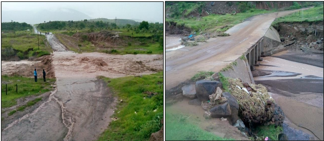
Figure 3: Examples of photographic evidence of hazards collected during site visits
